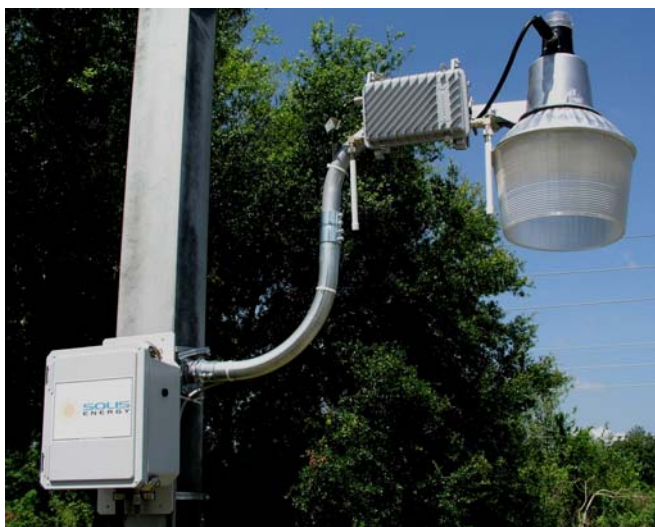
Solis Energy's 12030 Series AC>DC UPS and Streetlight Power Tap Adaptor combined to power WiFi radio.
